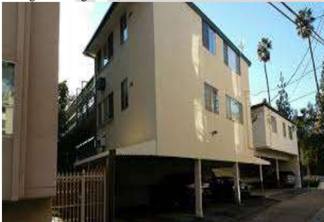
Fig. 1.1: Building with soft storey
