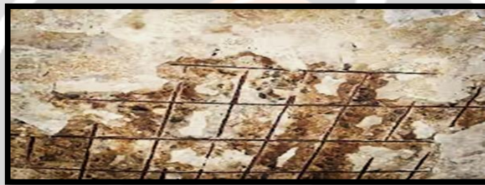
Figure. 2 Reinforcement corrosion on water tank
