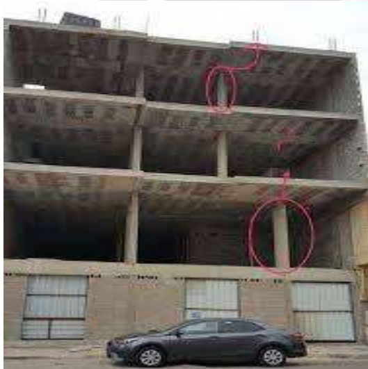
Fig 1.1 :Structure showing Floating Columns
