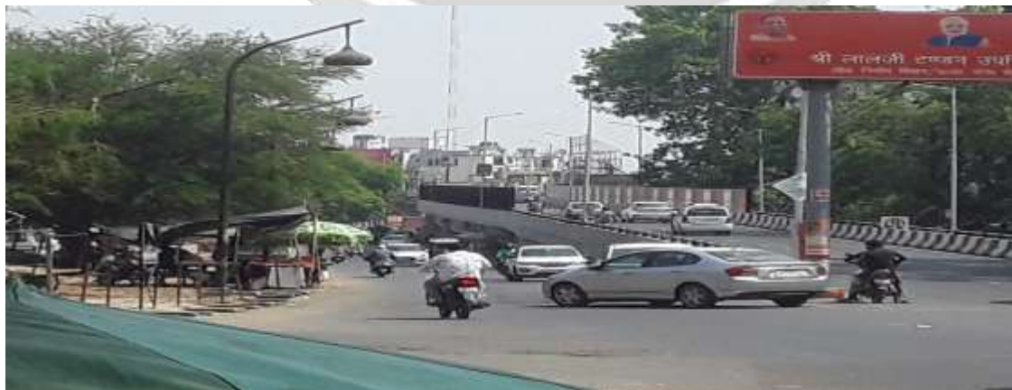
Fig 3. Image of Tulsidas marg flyover
