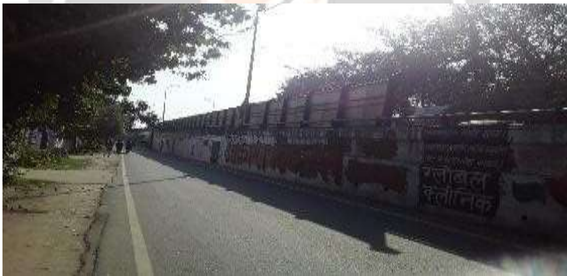
Fig 5. Image of Nirala nagarmarg flyover
