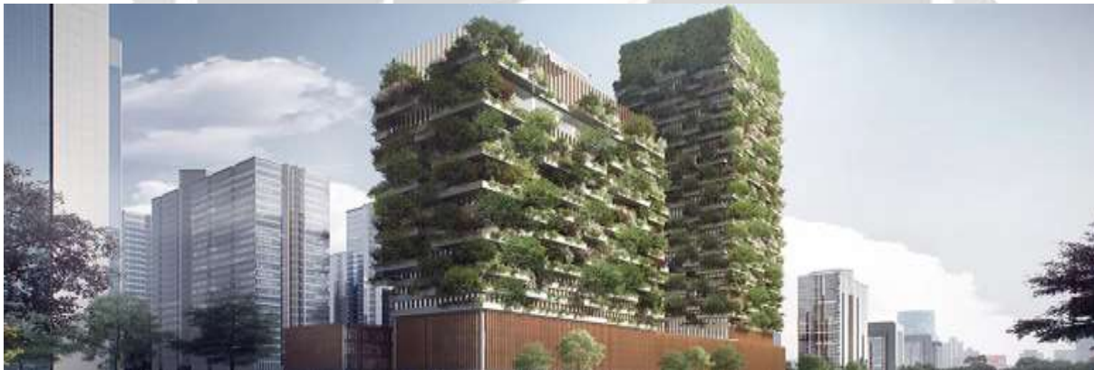
Fig – 4: Nanjing Vertical Forest https://wfmmedia.com/wp-content/uploads/2022/03/Green-Buildings.jpg
