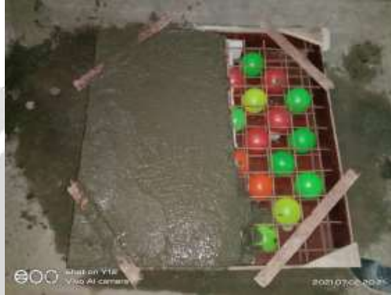
Fig.10: Partially Casted Model Bubble Deck Slab
