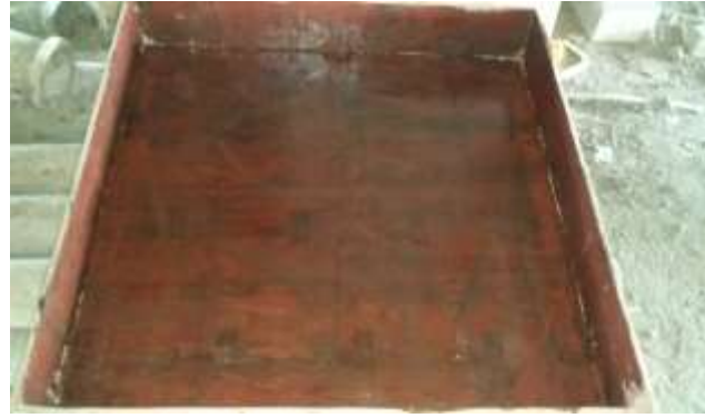
Fig.7: The material used for shuttering are boards (Formwork)
