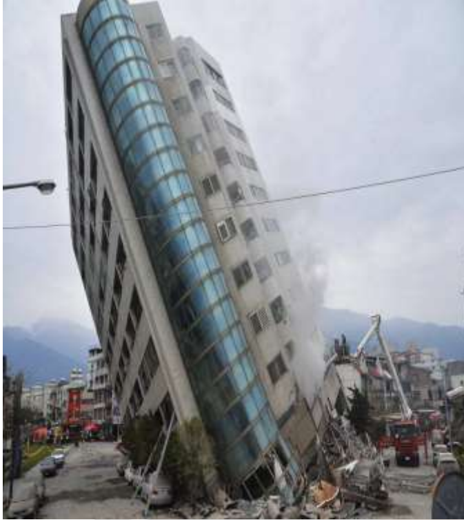
Fig. 1.1: Collapse of building due to earthquake
