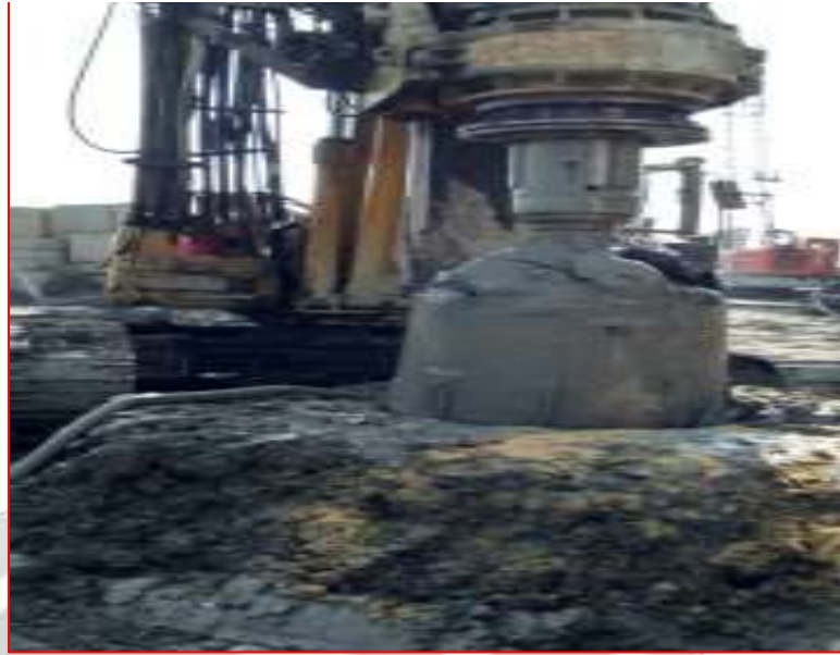
Figure-1 Rig fitted with auger on work (boring)
