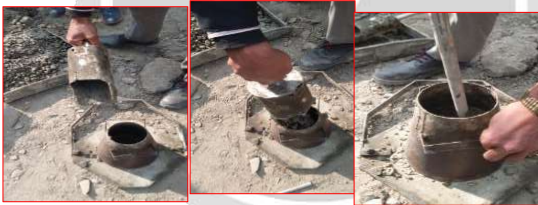
Figure-5 Slump test carried for concrete
