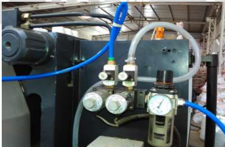
Figure:- Pressure Testing & Leakage Testing Of Product On FRL Unit.
