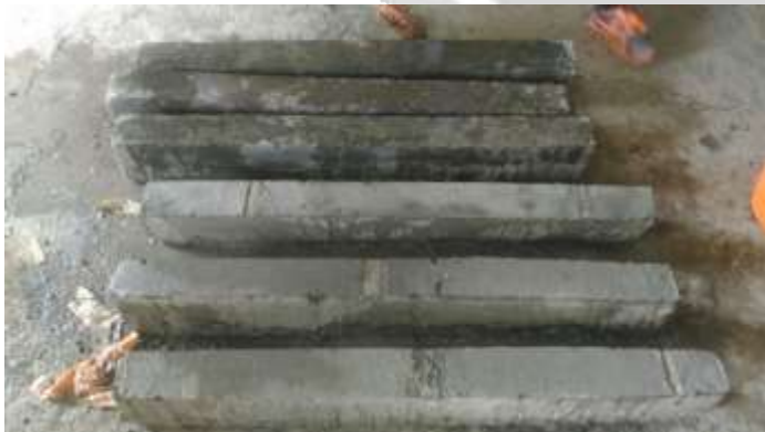
Fig.2- Beams after removal of formwork
