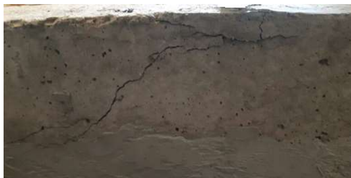
Fig.5- Shear Cracks in Beam B8
