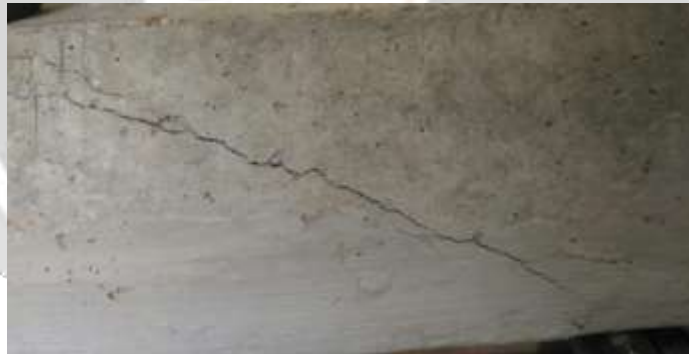
Fig.4- Shear Cracks in Beam B4
