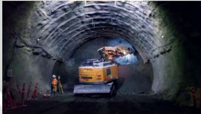
Fig -1 Excavation of the Tunnel
