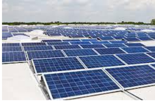
Fig-1: Solar Panels
