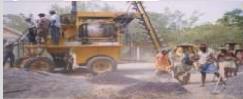
Fig. 9 Road construction using plastic waste [10]
