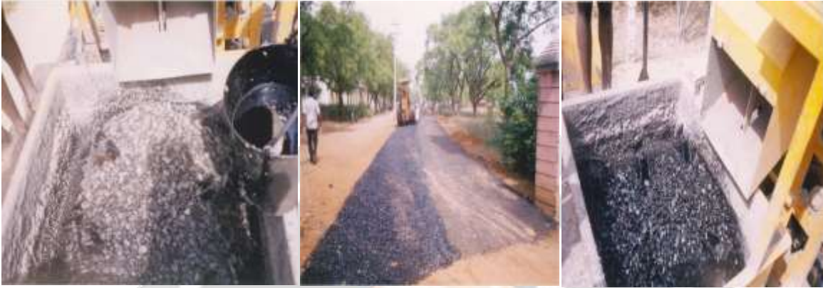
Fig. 11 Laying of plasticated road [11]
