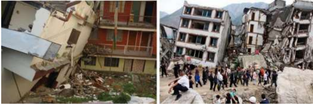
Figure 1.1 Typical failure of RC buildings in past earthquakes
