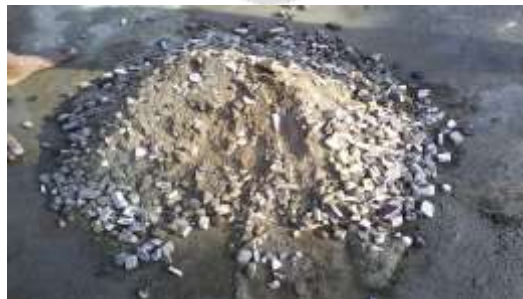
Fig:5 Mixing of Concrete
