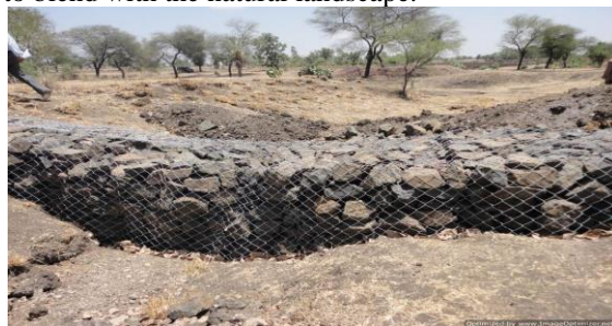
Fig-2- Gabion Structures
