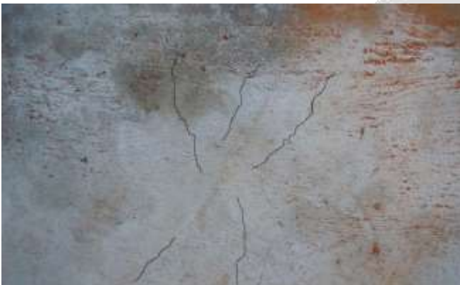
Fig - 7: shows the cracks form on SFRC
