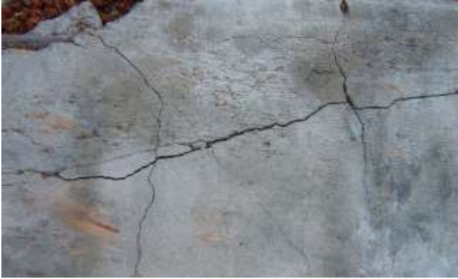
Fig - 6: shows the cracks form on NRC
