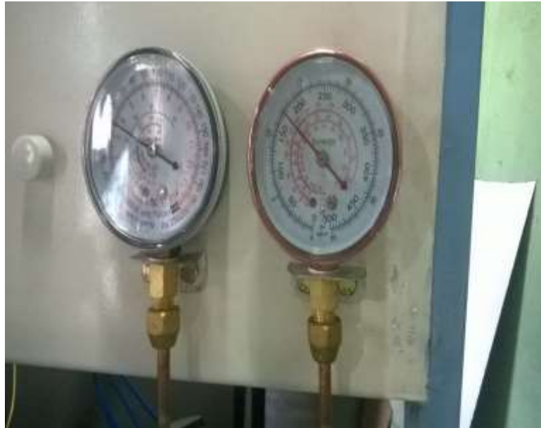
Fig. 4.1- pressure and compound Gauge
