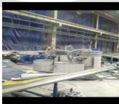
Fig. 5.1- Working without improper suction
