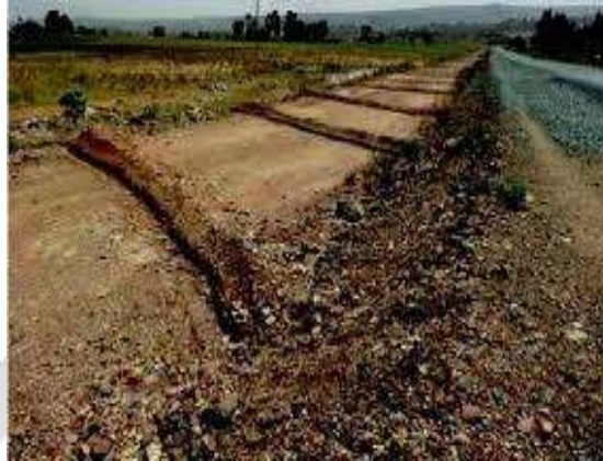
Fig.2.: Spreading Water from Road Surface and Culverts into Farmland
