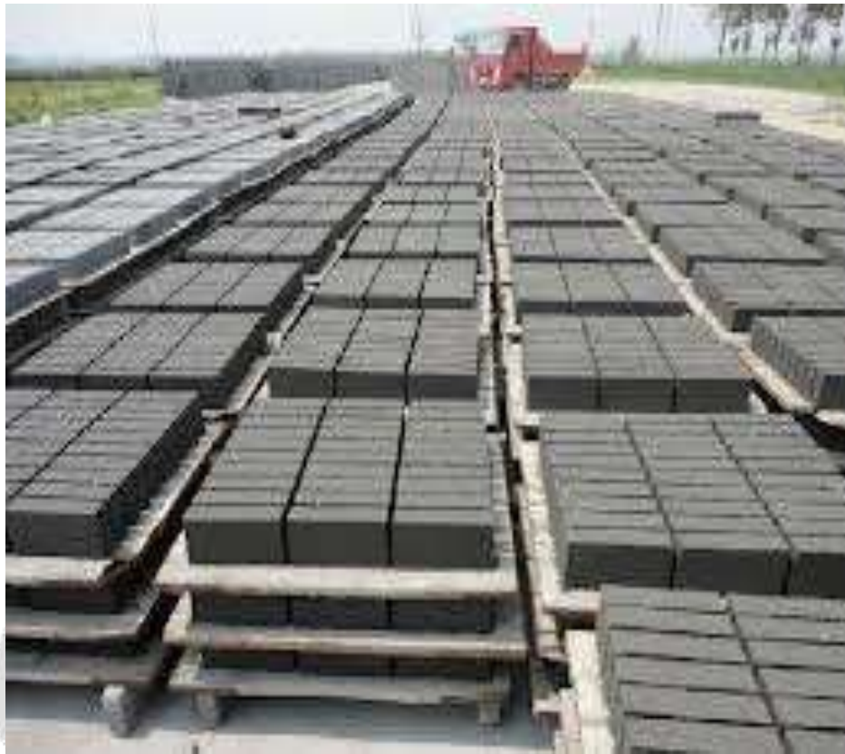
Fig. 1 Placing Hollow Concrete Blocks
