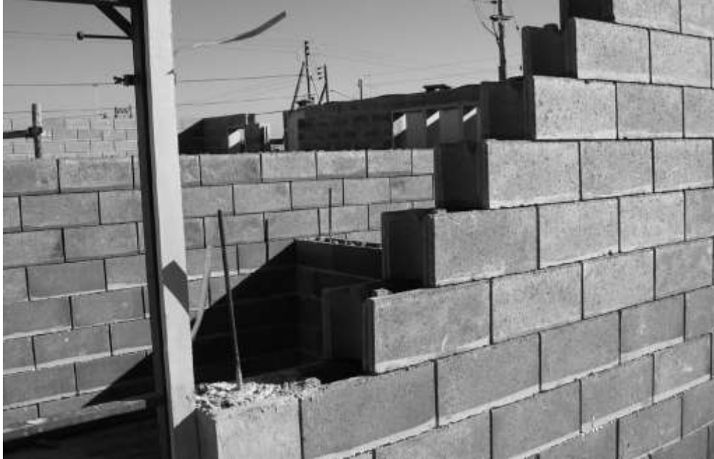
Fig. 6 Hollow Concrete Block Wall
