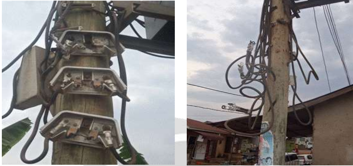
Photo 1: Protection status of distribution transformers on the LV side
