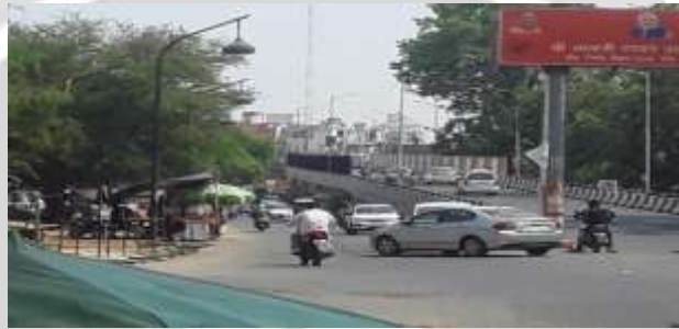
Figure 3. Tulsi Das Marg Flyover
