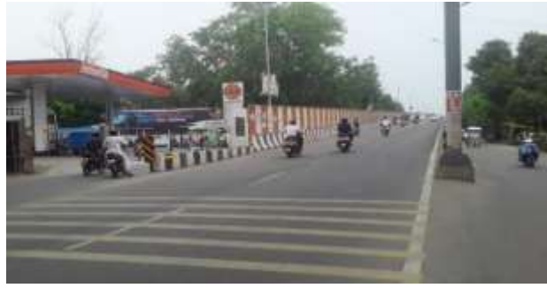
Figure 2. Talkatora Road Flyover
