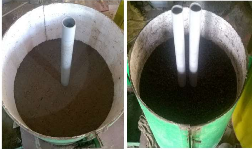
Figure- 2: Installation of single and twin fly ash columns
