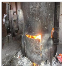
Fig -4 : Burner of the pyrolyzer prototype
