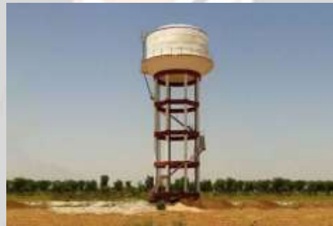
Fig 1.1: Elevated water tank
