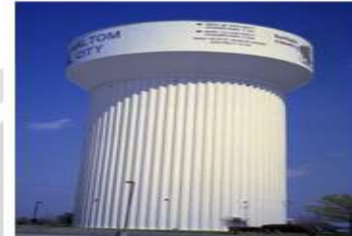
Fig 1.2.3: Elevated water tank
