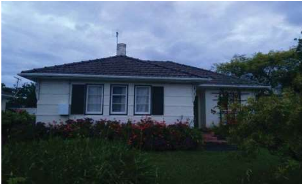
Fig. 1 (B). The building installed with the Smart Aging system
