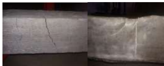
Fig 8 View of visible crack on the control specimen and retrofitted beams
