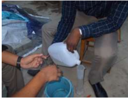
Fig 2 Mixing of epoxy resins
