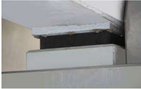
Fig -3 Elastomeric Rubber Pads Isolator
