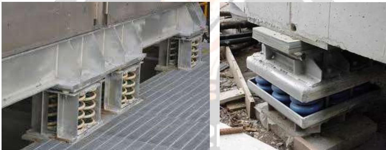
Fig -6 Spring Isolation System
