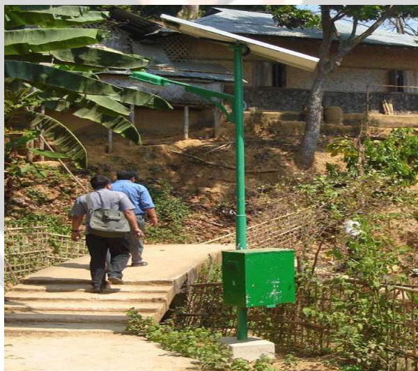
Fig. 2: Solar PV powered Street light at Barkal Upazila under Rangamati District.
