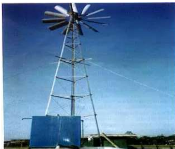
Fig. 4 shows a photograph of wind pump system set up by Bangladesh Centre for Advanced Studies at Patenga, Chittagong, Bangladesh [17]
