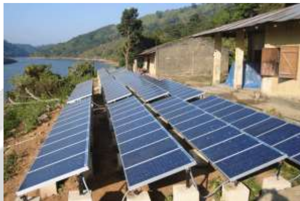
Fig. 1: Centralized AC Market electrification system at Barkal upazila under Rangamati District.
