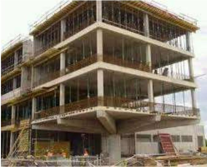
**Fig. 2: A multi-story at site with floating column**
