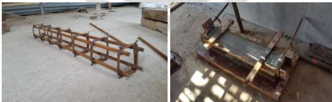
Fig-1 Casting of RCC beam
