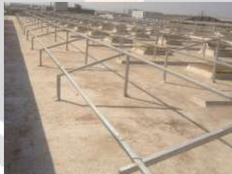
Fig. 4.1: Galvanized Iron Structure [4]
