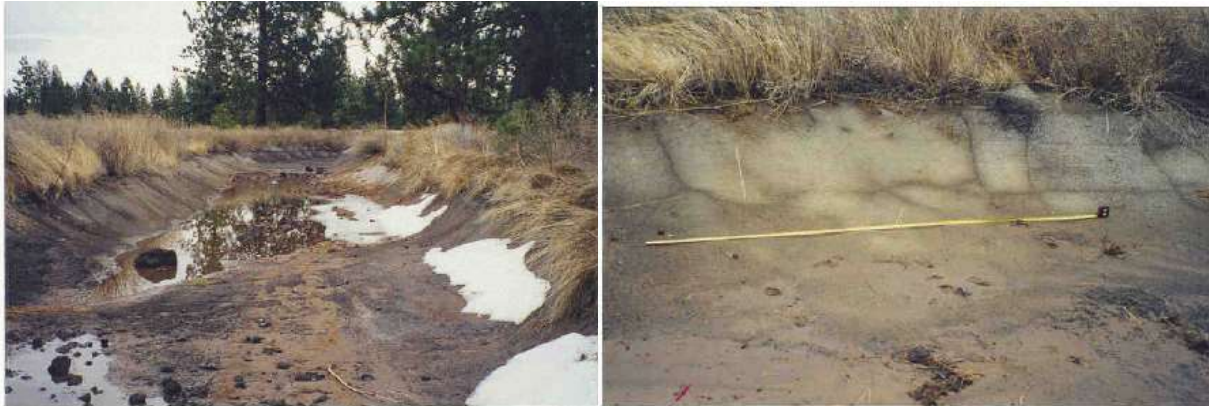
Fig -3: Lining using Shotcrete
