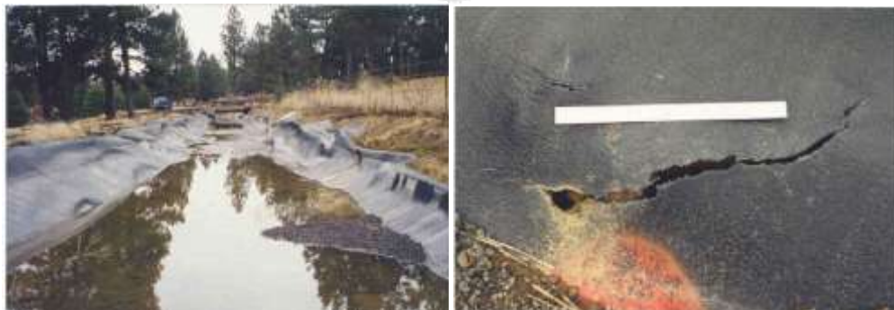
Fig -4: Lining using Exposed HDPE sheet
