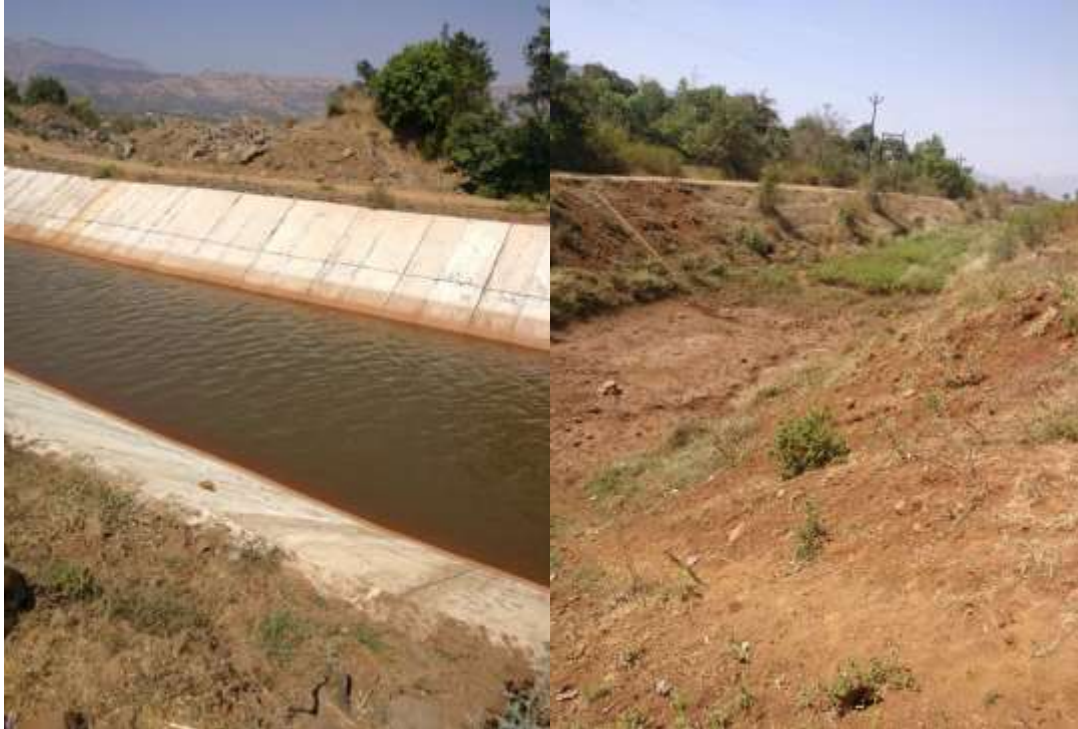
Fig -2: Canal condition of Nira Deoghar (Lined and Unlined)
