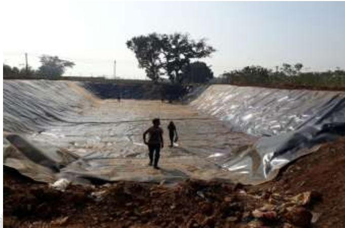
Fig -6: HDPE sheet after laying
