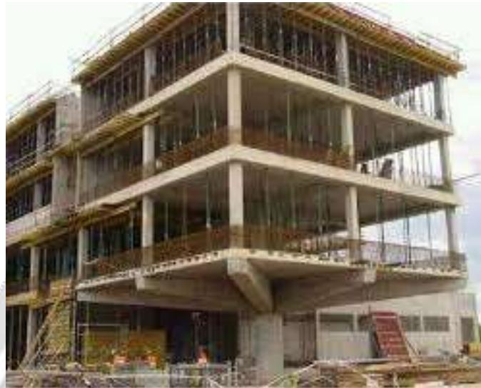
Fig. 2: A multi-story at site with floating column
