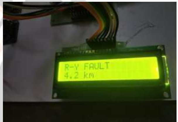
Fig -5: L-L Fault
