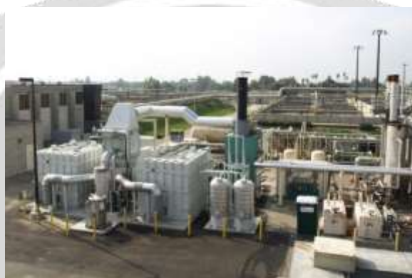
Figure 9: World's Largest Biogas Fuel Cell Power Plant, California, USA.
