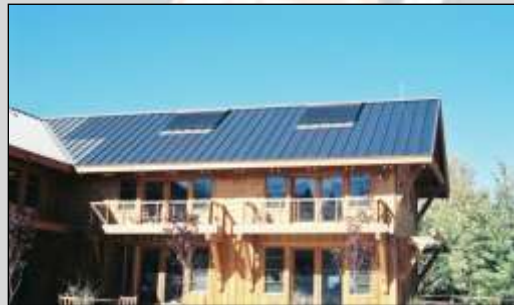
Figure 2: Solar Photovoltaic cover the roofs of an increasing number of homes.
