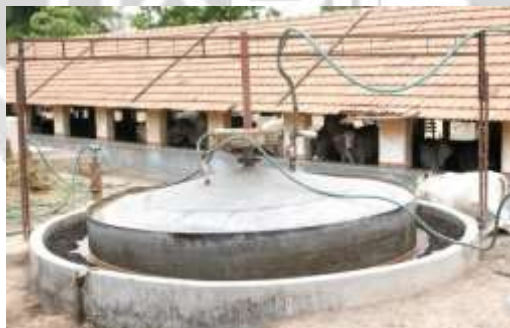
Figure 7: A typical Gobar gas plant.
