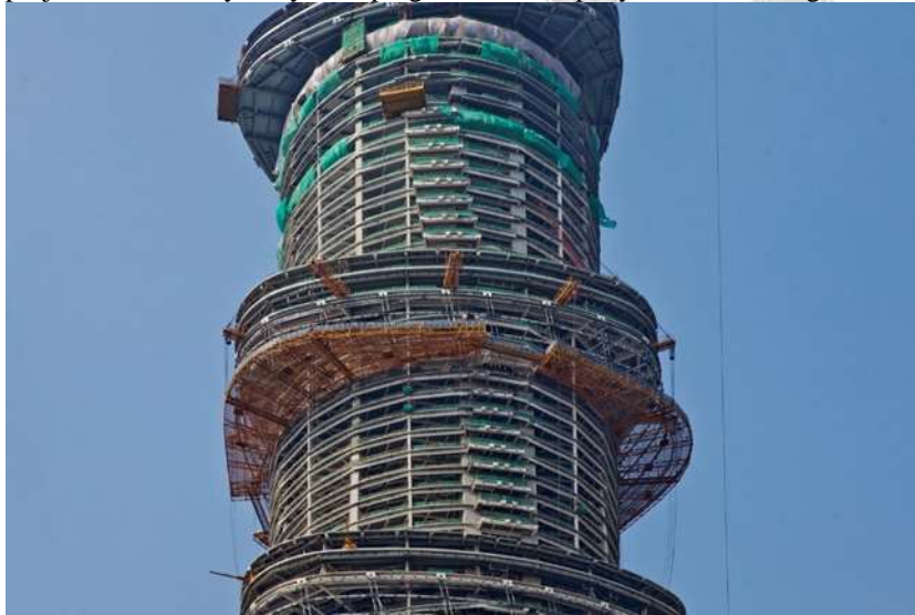
Figure 28 –construction of shanghai tower (Ardit, Nayak, & Damci, 2017)
