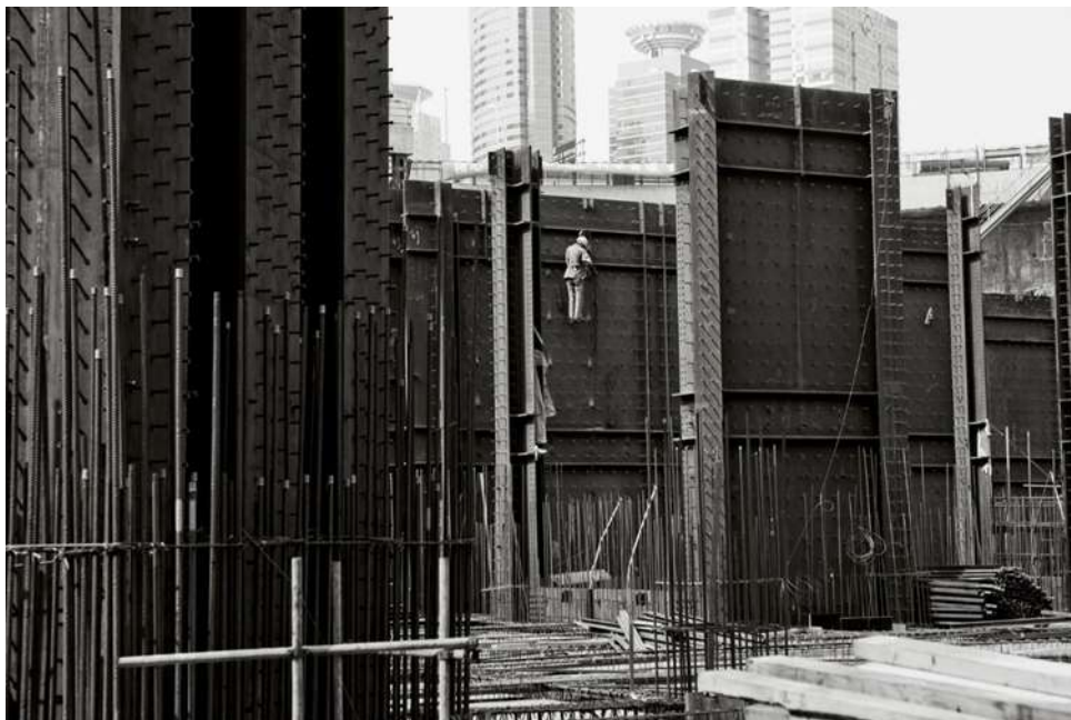
Figure 26 –During construction of shanghai tower (Ardit, Nayak, & Damci, 2017)
