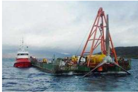
Fig.5 Hammerfest Strom horizontal-axis turbine being deployed in demonstration project, Northern Norway, 2003
