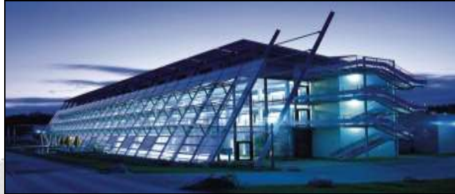
Fig -13: Building Integrated Photo - Voltaic Glazing [58]
