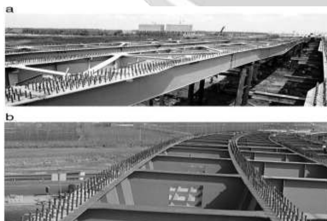
Fig 1.2 : Construction Picture of Composite Girder
