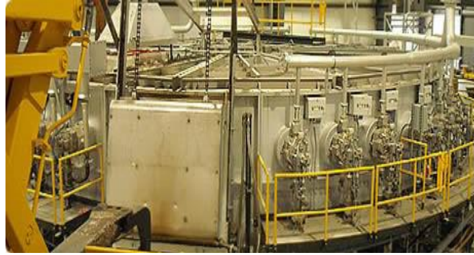
Fig -1: Normalising furnace
