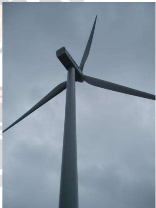
figure 2.2 Horizontall axis wind
