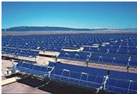
Fig.8 The SEGS CSS plant in San Bernardino County, California was built in the 1980s.
