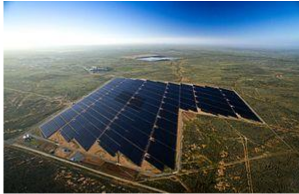
Fig.10 Broken Hill Solar Plant, New South Wales
