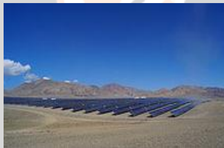
Fig.6 Present situation in A solar power plant in Russia
