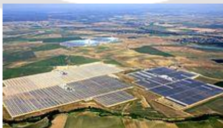
Fig.7 The first three units of Solnova in the foreground, with the two towers of the PS10 and PS20 solar power stations in the background.
