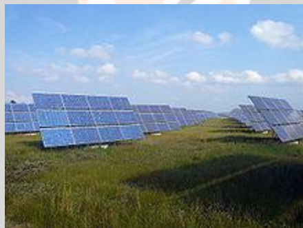
Fig.5 Present situation in Erlasee Solar Park
