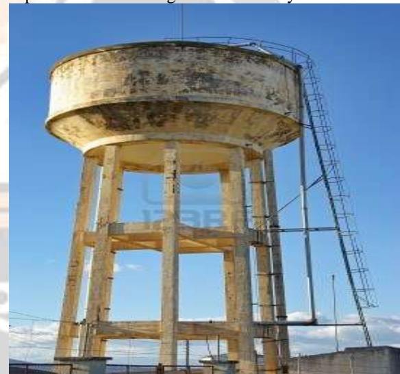
Fig -1: Elevated water tank supported on staging
