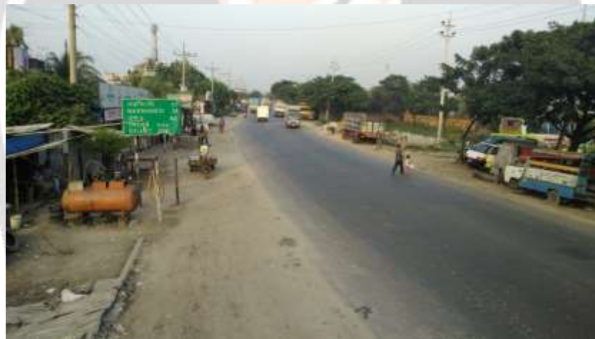
Fig-2: Tarabo Rupgonj Lane
