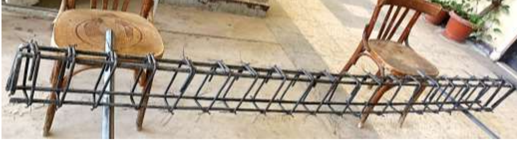
Fig.3: Steel reinforcement for beams
