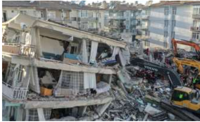
Fig 1.1 : showing column damage during earthquake excitation
