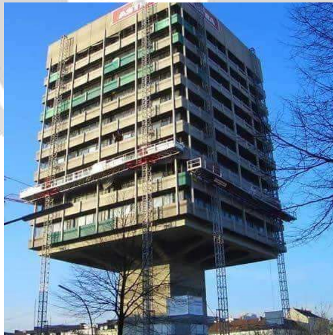
Fig. 1.2: Structure showing Floating Columns
