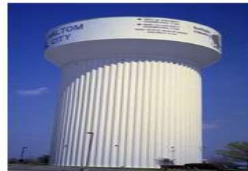
Fig 1.2.3: Elevated water tank
