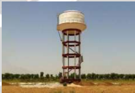
Fig 1.1: Elevated water tank
