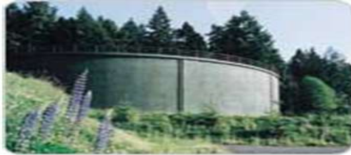
Fig 1.2: Ground water tank
