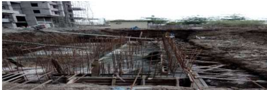
Fig.6 Form work and Reinforcement
