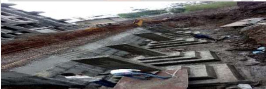
Fig.8 post concreting work
