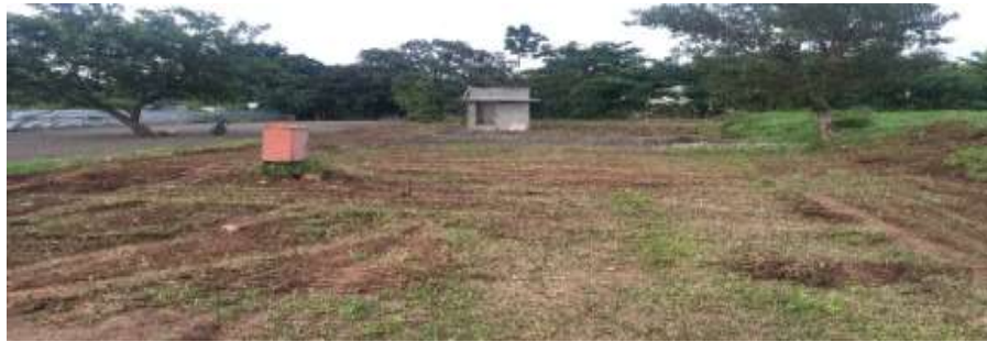
Fig.1 CQC cleaning for excavation
