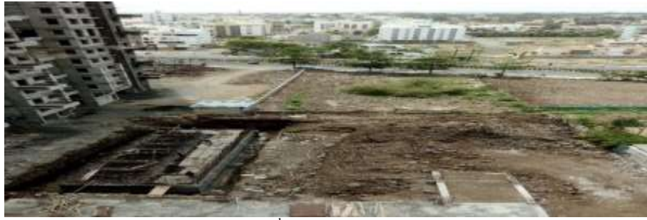
Fig.10 2 nd phase work of footing
