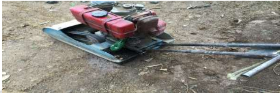
Fig.11 Compactor for dressing of base course
