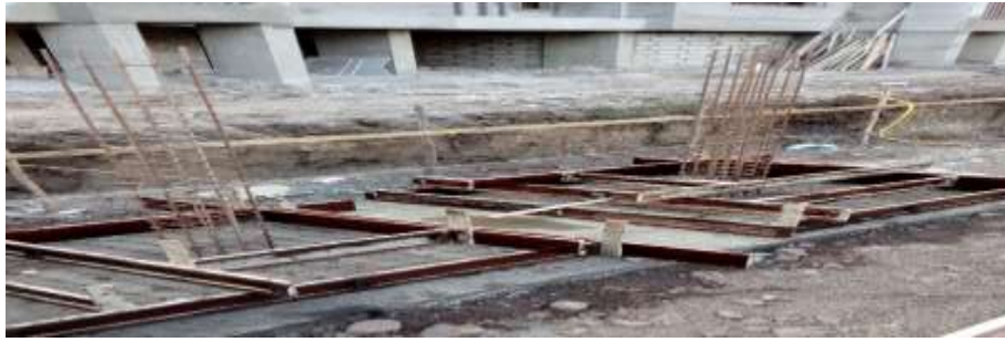
Fig.5 completed pcc work of Footing
