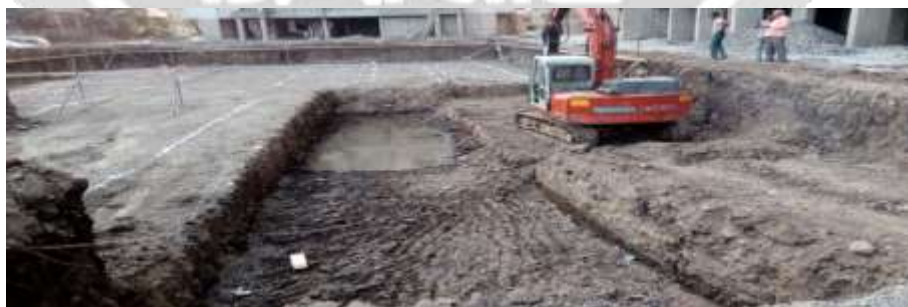
Fig.4 Excavation and dewatering work
