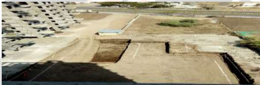
Fig.3 Dressed base course
