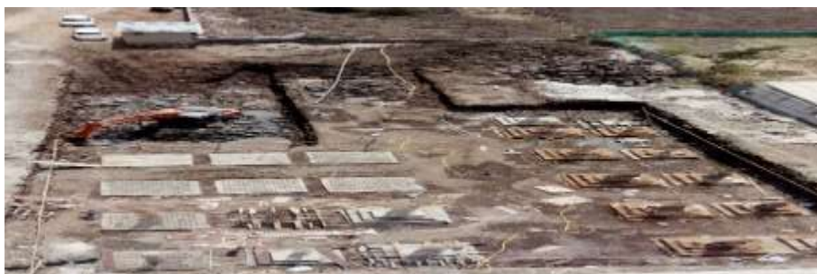
Fig.9 2 nd phase work of footing
